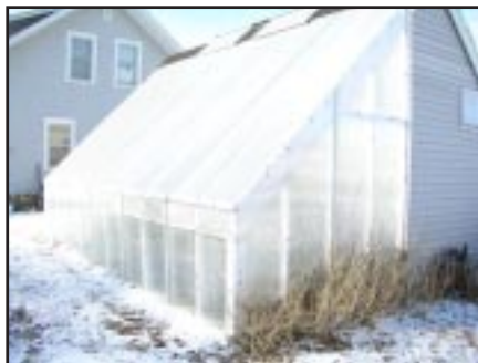
The extreme angle of the Garden Goddess greenhouse’s roof helps the building capture winter sunlight. (LSP photo)
