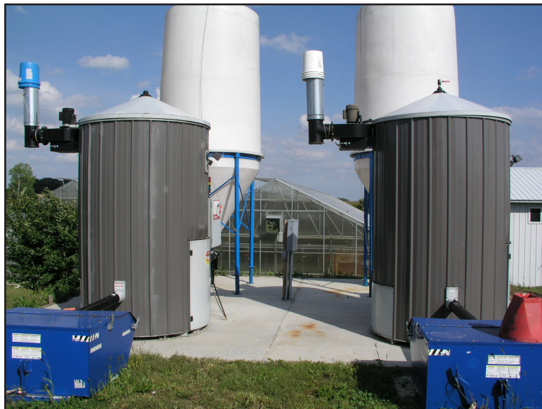
Two stoker furnaces on the Kreidermacher farm heat the greenhouses. The furnaces can burn a wide variety of plant material. (LSP photo)
